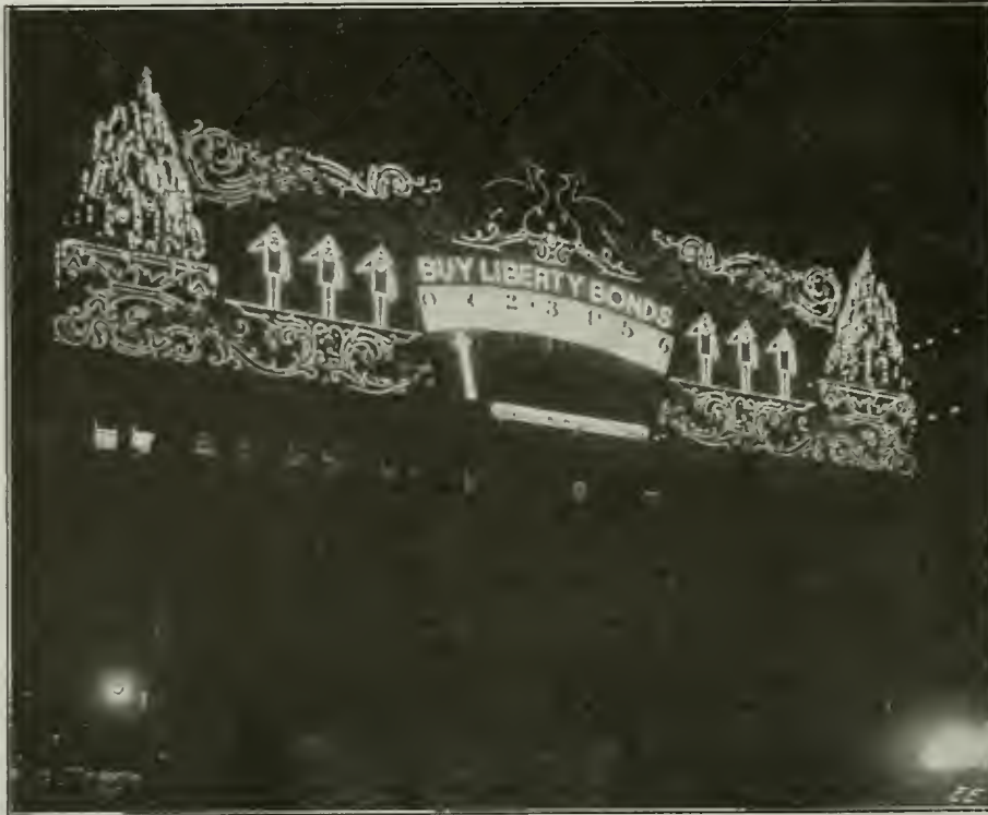
Spectacular Electric Sign One Block Long Which Kept Track of the "Fourth Liberty Loan" for New Yorkers. The Illuminated Needle Moved Slowly Across the Dial as the Loan Progressed.
