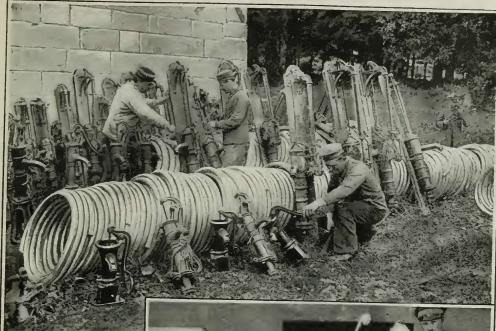
The battery of pumps above is used to draw the water out of a flooded trench. One motor pump would draw more water and in less time, and the German army is equipped with thousands of power driven pumps. Many of these hand pumps bear American trade-marks, and much of the piping was made in this country also
