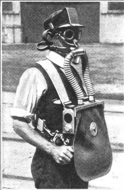
In the breathing bag oxygen and outside air are mixed
