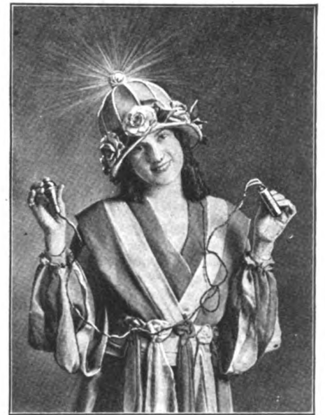
The lights are operated by a small dry battery, with push button
