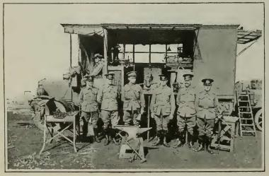
The great number of motor vehicles now in use in the war has necessitated the employment of vehicles whose sole purpose is to make quick repairs. The unit shown at the left is an American workshop with the Ninth Australian Corps. Note the complete equipment of forge, anvil, vise, drill presses and tools. Also note how the lower half of the body swings down to form a convenient working platform
