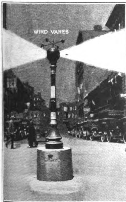
Small cup shaped vanes, rotated by the wind, operate this silent traffic policeman
