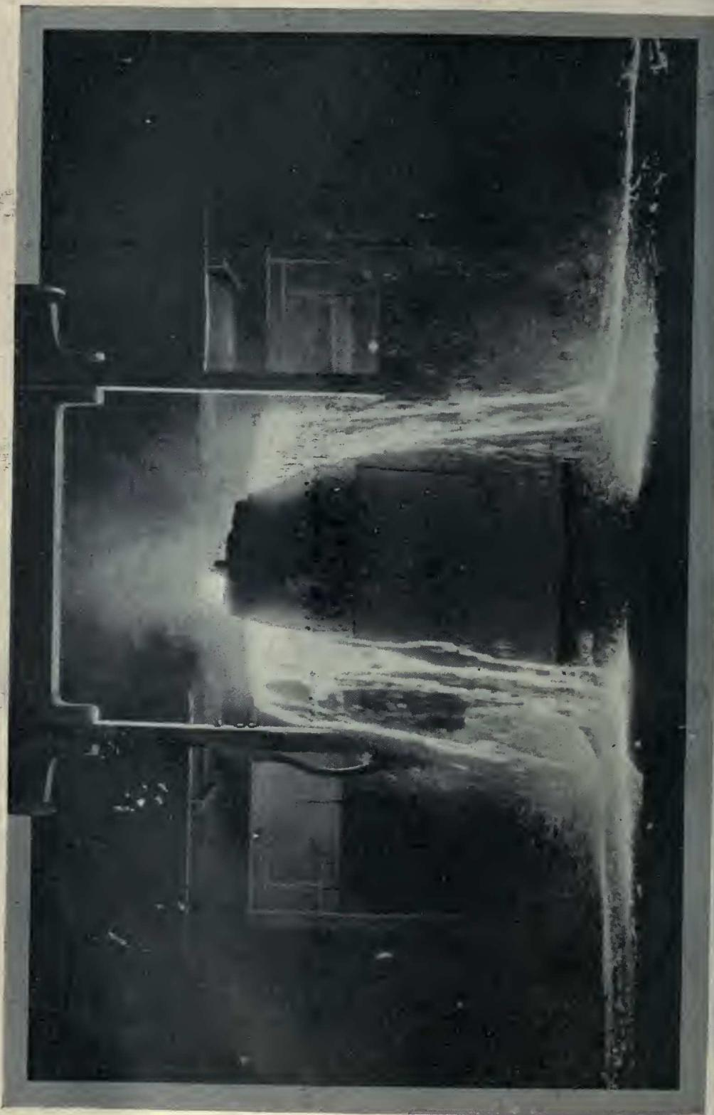
This photograph was taken by the light emanating from the incandescent molten metal out of which a modern monster gun is being made. The ladle carries fifty tons of the metal, which is allowed to overflow continually so as to remove superfluous impurities and slag automatically. The framework over and around the ladle is the electric hoist by which the immense weight is lifted and transported from one process to the next.
