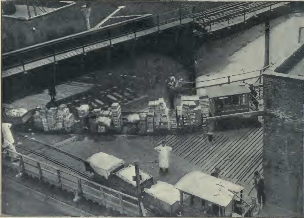
A miniature electric railway by means of which half a million pounds of meat are handled daily. Nine hundred cars, driven by seven electric locomotives are used in one packing establishment
