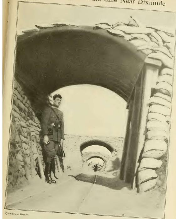
This peculiar series of bridges constitutes a protective measure that war conditions have evolved. The railroad is a narrow-gage line near Dixmude which is used for transporting supplies on low flat trucks by man-power. Owing to the liability to bombardment by airplanes, it was found necessary to provide shelters, for which reason these bridges were built at intervals as a protection for both men and cars. Compare with officer for height
