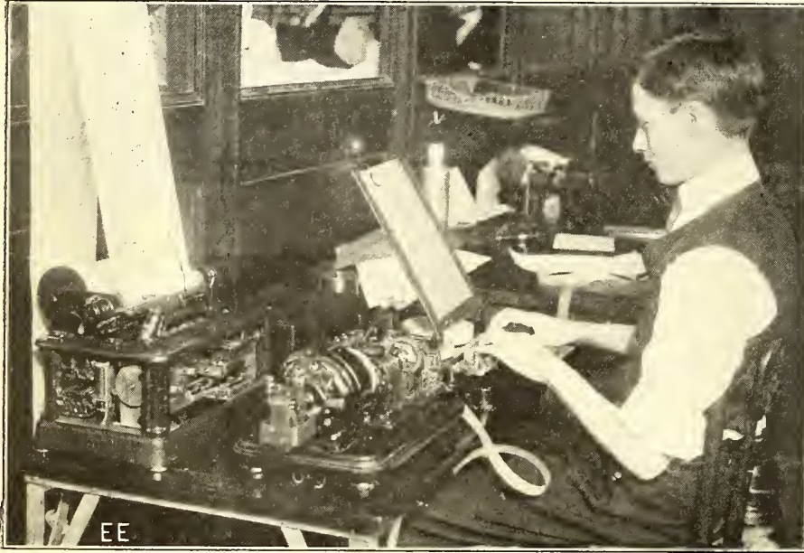
Photo (C) by Underwood & Underwood. Showing Morkrum Sending and Receiving Printing Telegraph System Installed in Associated Press Offices in New York City. Local Printer to Left.
