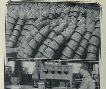
At left below: A twin machine that automatically turns two shell bodies at the same time to the right diameter. The shells being made are sixinch high explosive shells, used in the smaller naval guns and in field pieces
