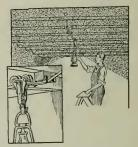
Instead of depositing the lantern on the floor, on an upturned box, where its light is usually shed to the least advantage, he has devised a simple but effective overhead trolley system. A stout wire is extended across the ceiling between braces, and the lantern suspended on a small wheeled truck from it.
