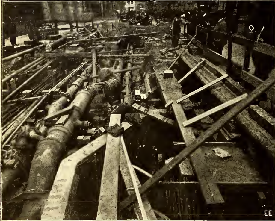
Showing Vast Net Work of Electric Gas, Water and Steam Conductors in a New York City Street Exposed During Building of New Subway.
