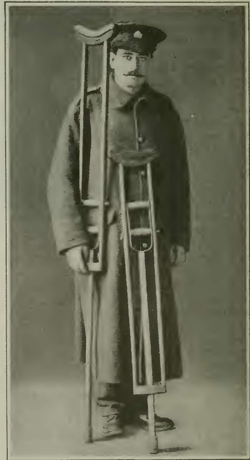
The Germans made these adjustable crutches to be used by long and short men
