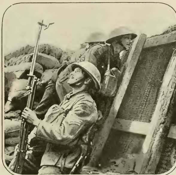
By attaching an ordinary trench mirror to the end of his bayonet blade the Tommy has a makeshift periscope
