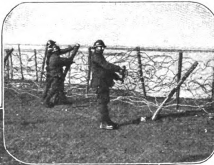
Italian troopers erecting a barbed wire entanglement along the Piave. Wire stretchers are used very much like those with which our Western ranchmen are familiar
