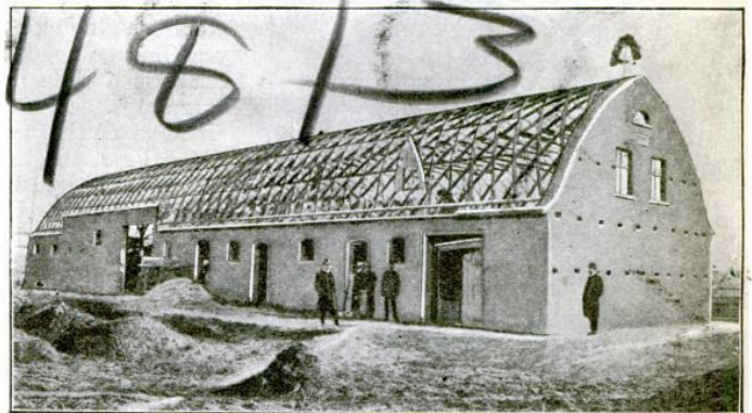
A molded house nearing completion. Note the roof construction
