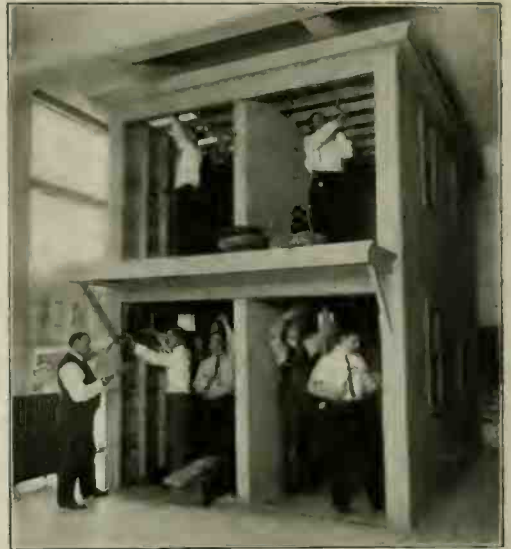
Training Future Electricians in a Miniature House in Which They Drill Beams, Put Up Cleats, Run Conduit, and Perform All the Other Tricks of the Trade Which the Practical Man Must Learn.
