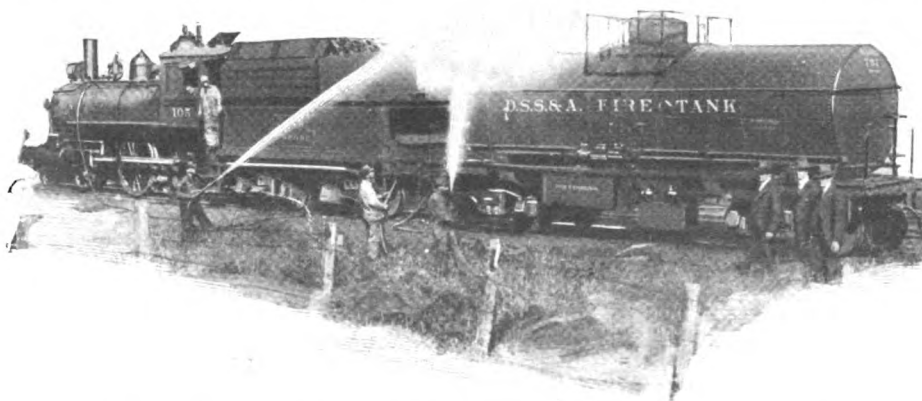
A forest fire near the railroad tracks? This converted oil-tank will race to the scene. It is filled with water now and has two powerful pumps
