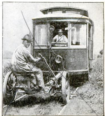
Mowing weeds along the right of way
