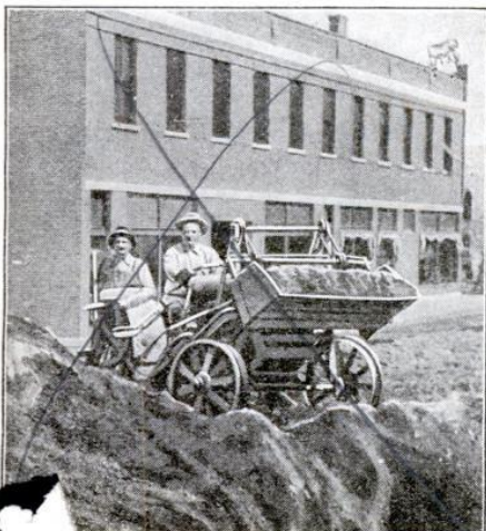
Power shovel used for excavating
