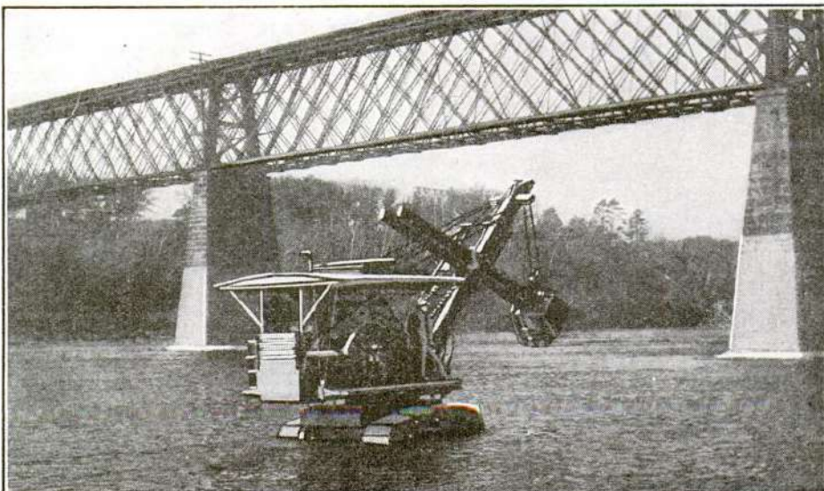
The amphibious excavating shovel in midstream, bucking the current under its own power
