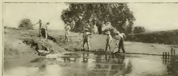
The saw, from 150 to 300 feet long, cuts the weeds; a wooden grating collects them and a rake removes them
