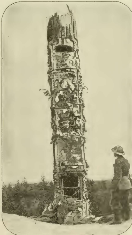
A three-storied German observation post constructed within the hollow of a tree
